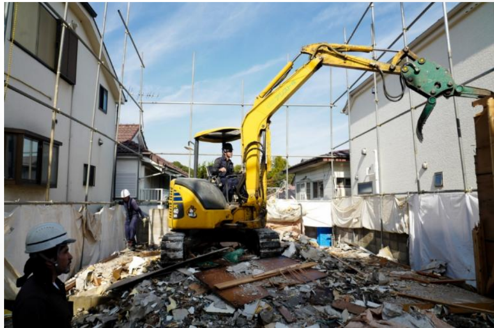
Warabii:2017. Kurdish workers are working for construction and demolition companies
